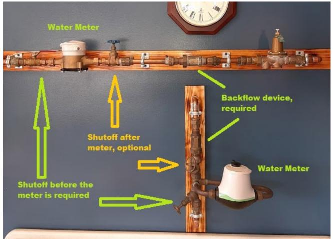
Shown above two, a Horizontal setup, and a Verticle setup utilizing a K-Horn
